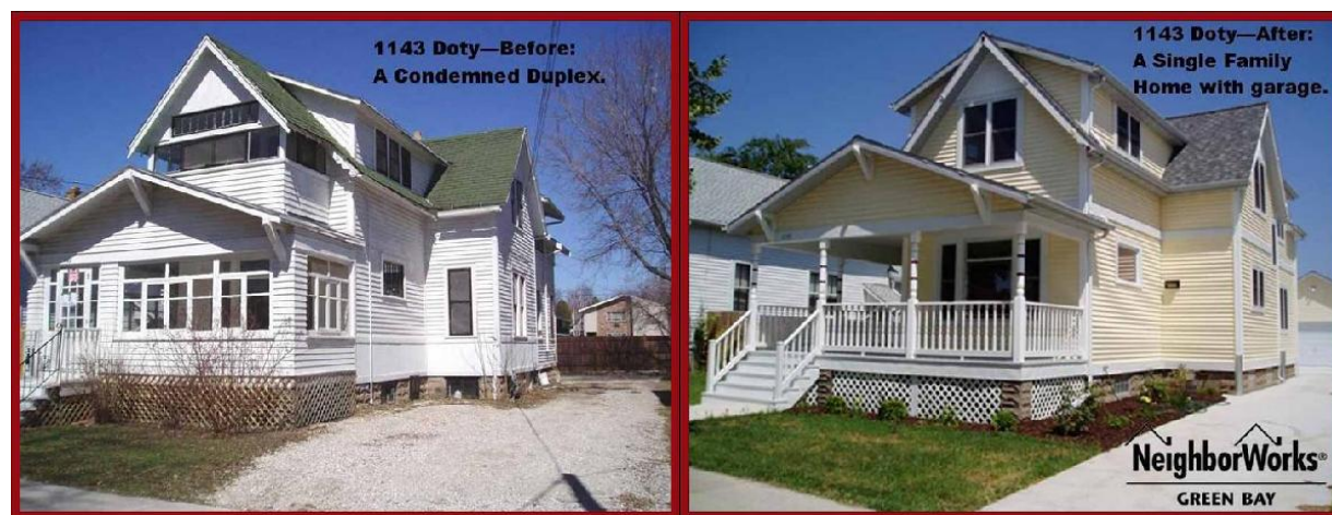
Example of before and after housing renovation by NeighborWorks Green Bay
